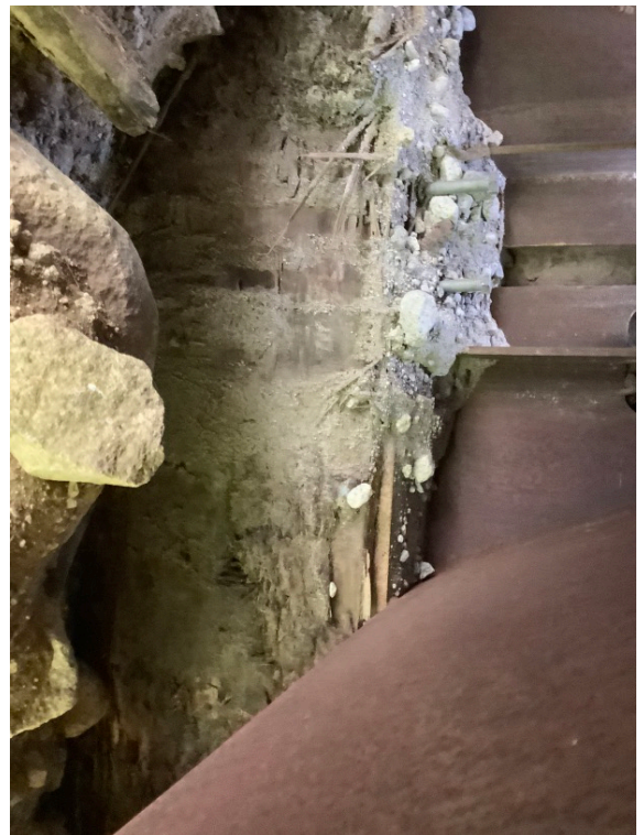
Left Bank Abutment when facing downstream
